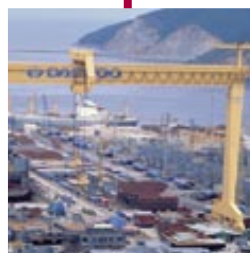
SHIPYARD CRANES feature a comprehensive range of jib portal and Goliath gantry cranes.
