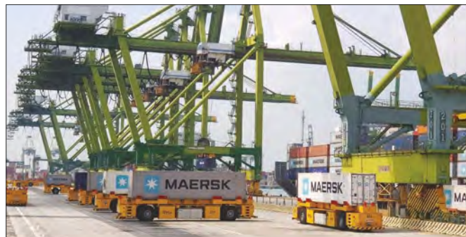
After six years of testing, PSA has decided to use transponder technology for AGV navigation at Tuas Mega Port
