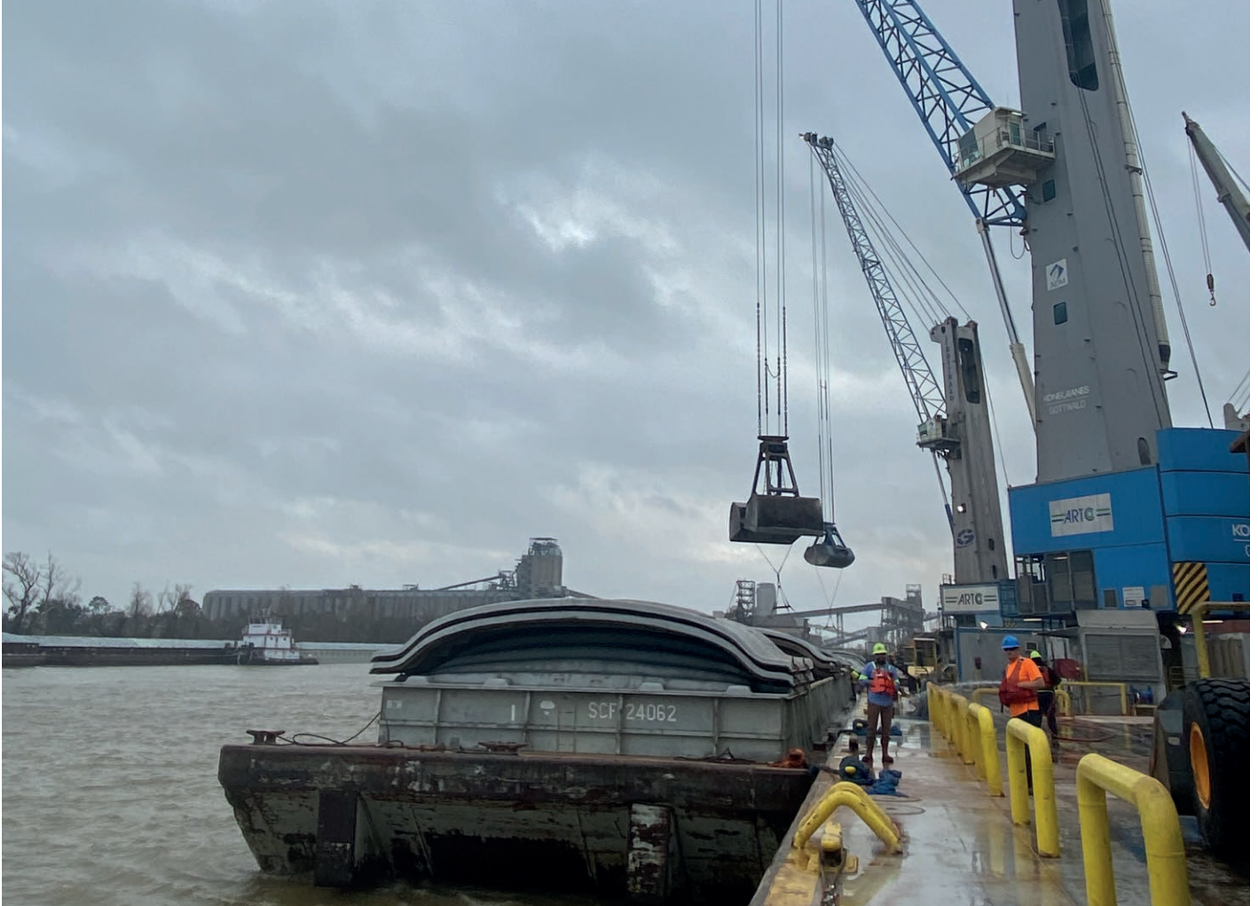
The first-time retrofit on one of the ARTCO floating cranes in the lower Mississippi simplifies maintenance with improved parts availability. Photo Courtesy of ADM
