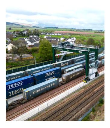
Fully electric operation requires less maintenance, produces less noise and reduces emissions. These are particularly important considerations if your container terminal is near a residential area.
