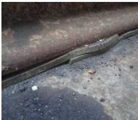
Rail pad not properly installed.
