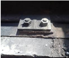
Rail clamp welds starting to corrode.
