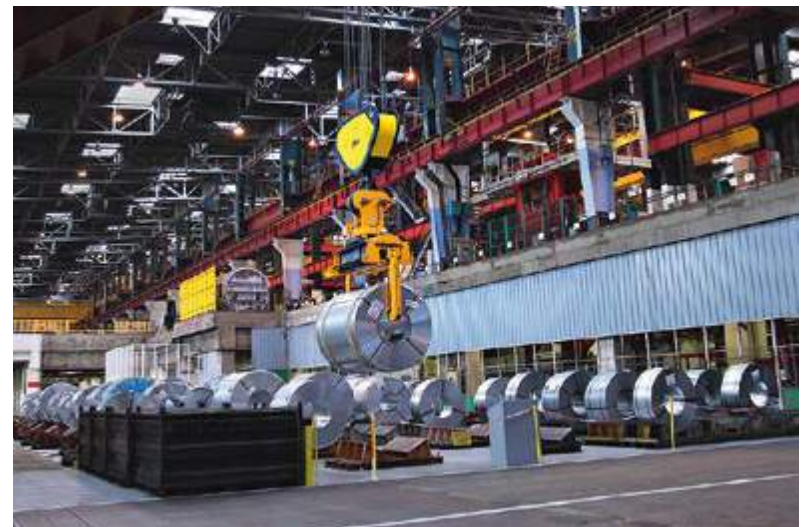
Renault trusts Konecranes to move its steel coils safely and efficiently at its factory in Sandouville, France.
